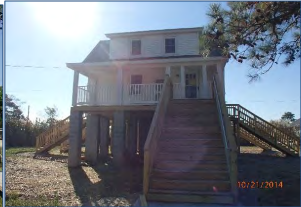
Figure 76: House in Hayes, Gloucester County - AFTER elevation.
