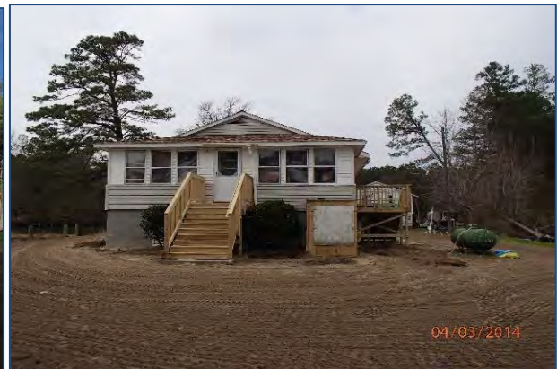
Figure 78: House in Hayes, Gloucester County - AFTER elevation.
