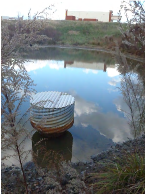
Figure 1: Wet pond with metal overflow structure
