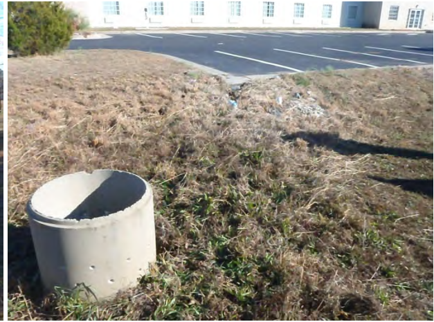
Figure 2: Riser structure at northern end of basin
