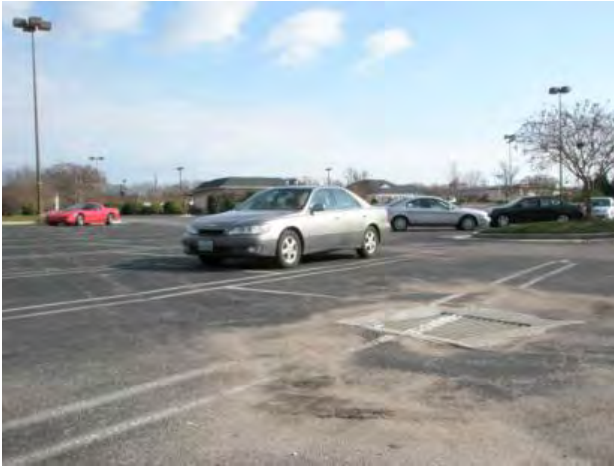
Figure 1: Typical parking lot inlet
