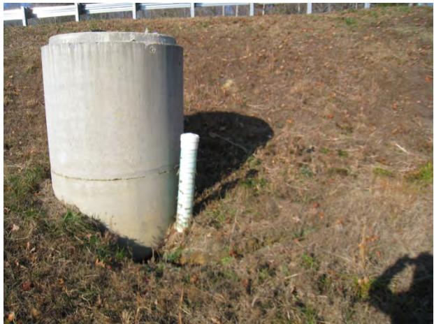
Figure 4. Basin outlet, with erosion at base
