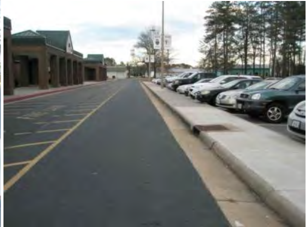
Photo 2: Driveway drainage to Biofilter B
