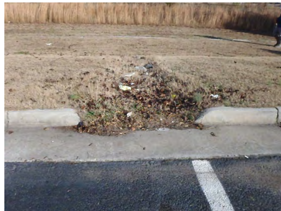
Figure 3: Partially clogged inlet to basin
