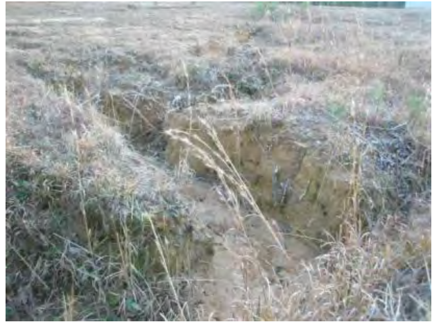
Figure 2: Erosion of outlet
