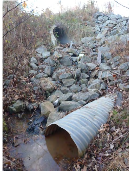
Figure 2: Metal outlet pipe partially clogged
