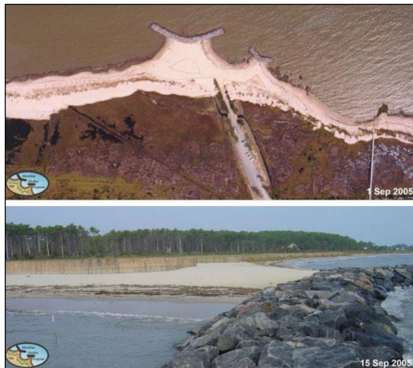
Figure 11 - Aerial photo (top) and ground photo (bottom) taken at Haven Beach after breakwater and beach fill installation in 2005.
