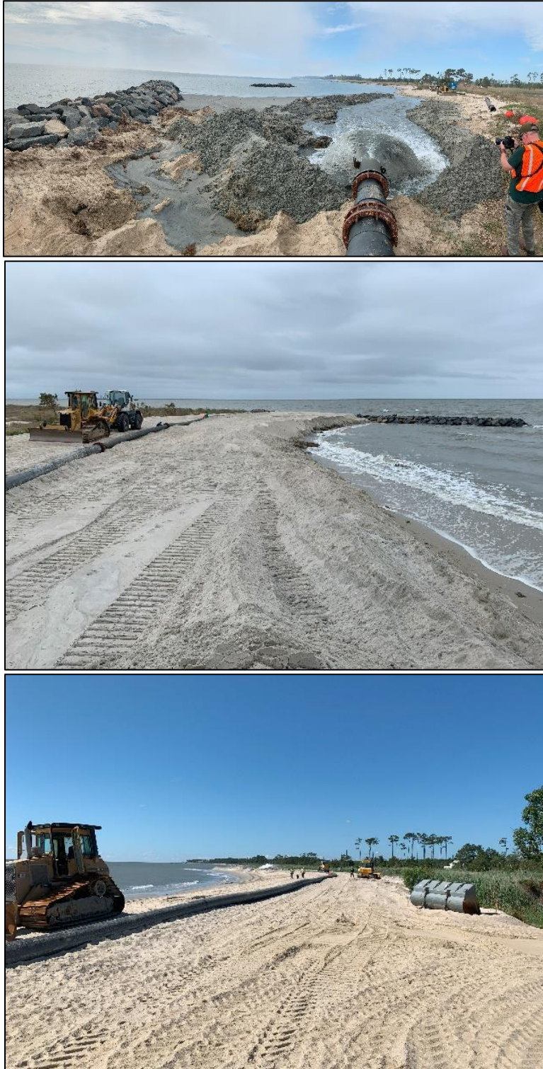
Figure 12 - Construction of the first breakwaters and living shoreline at Haven Beach (2024).
