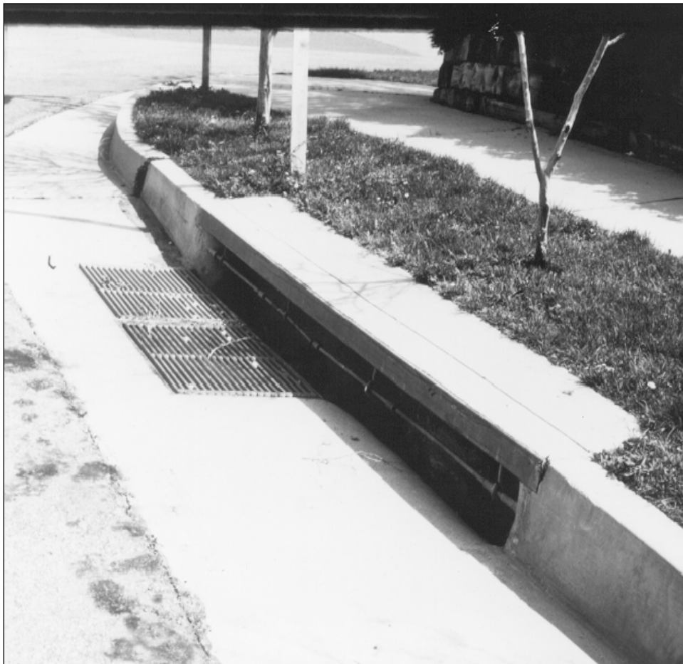
Figure 7.12. Sweeper combination inlet.
