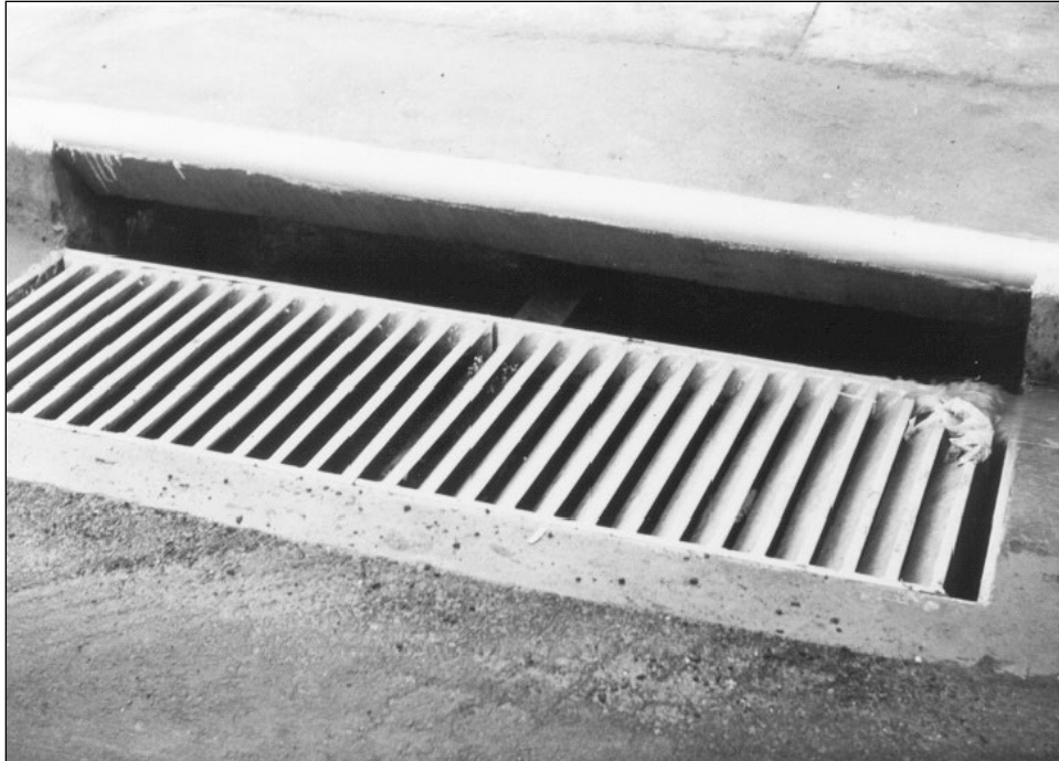
Figure 7.11. Combination curb-opening with 45-degree tilt-bar grate inlet.
