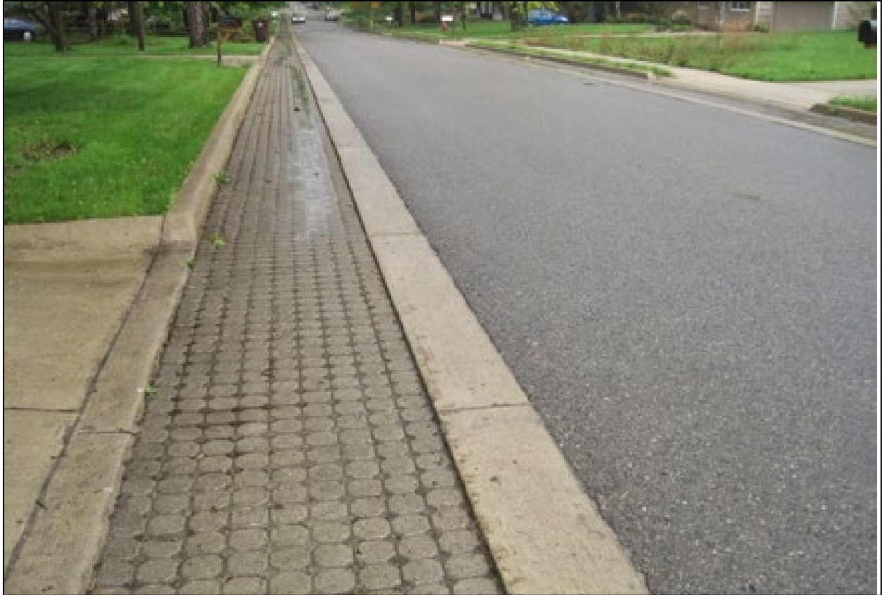
Figure 11.10. Green infrastructure practice: permeable pavers (USEPA 2021).
