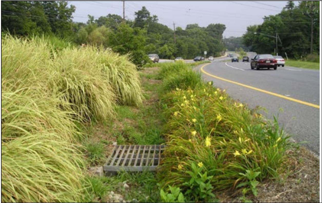
Figure 11.8. Green infrastructure practice: bioswale (USEPA 2021).
