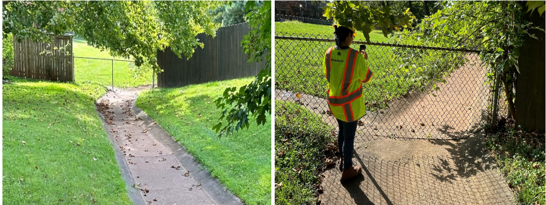
Figure-10: A wood fence and a chain link across the stream and the flood plain constructed by a homeowner, which might increase the flood hazard.
