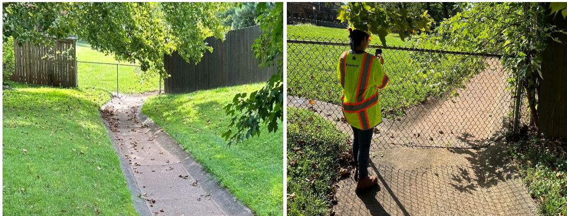
Figure-10: A wood fence and a chain link across the stream and the flood plain constructed by a homeowner, which might increase the flood hazard.
