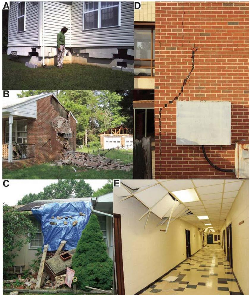
**Figure 25: Examples of Structure Damage in Louisa County, Virginia After the 2011 Earthquake<sup>76</sup>**
