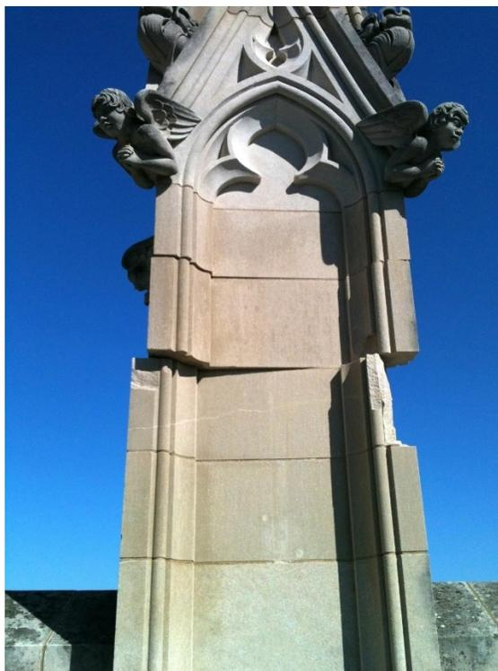
**Figure 26: Earthquake Damage to Washington National Cathedral in Washington, D.C. After the 2011 Earthquake<sup>77</sup>**
